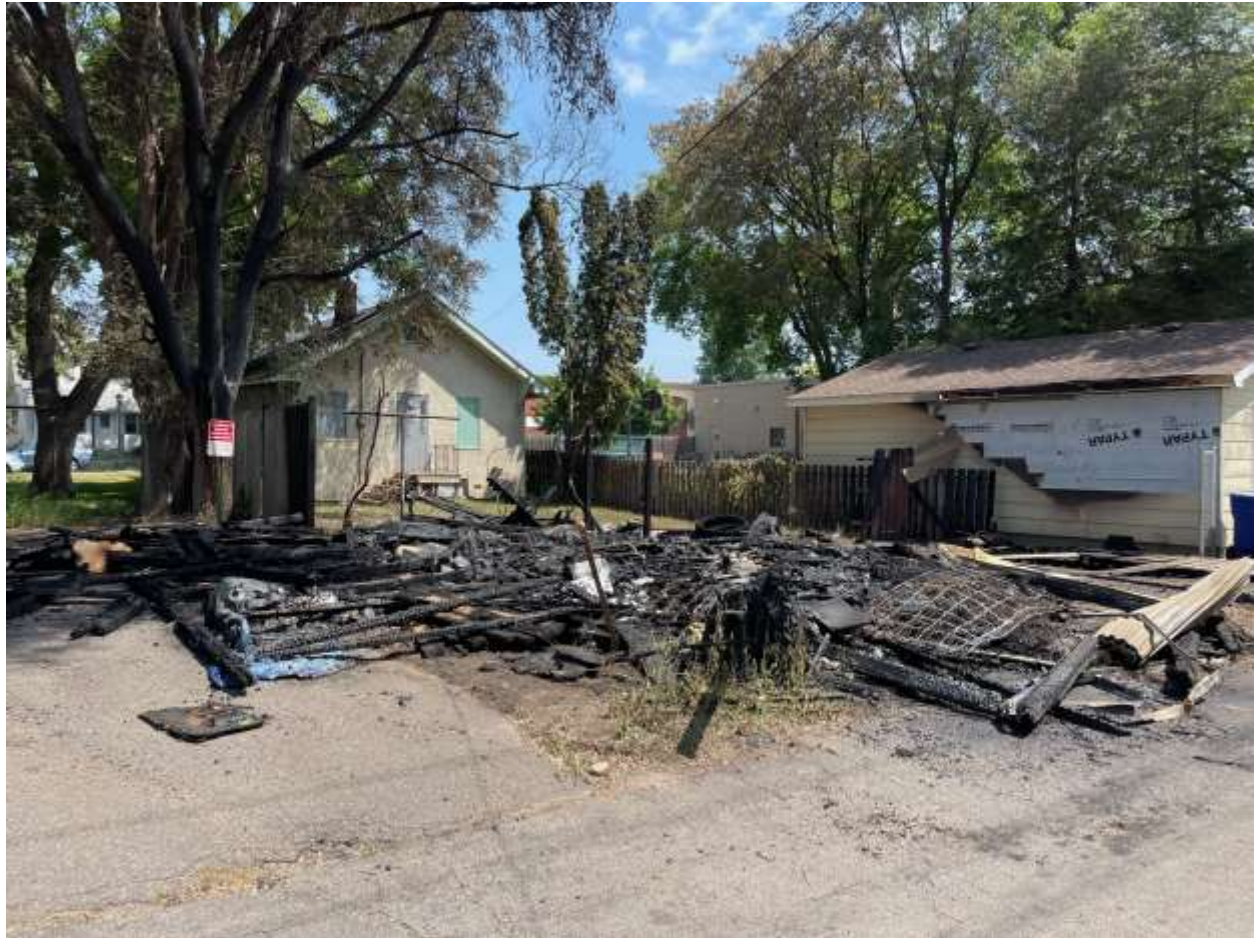
792 Rose Ave E. Garage fire 6/28/23
