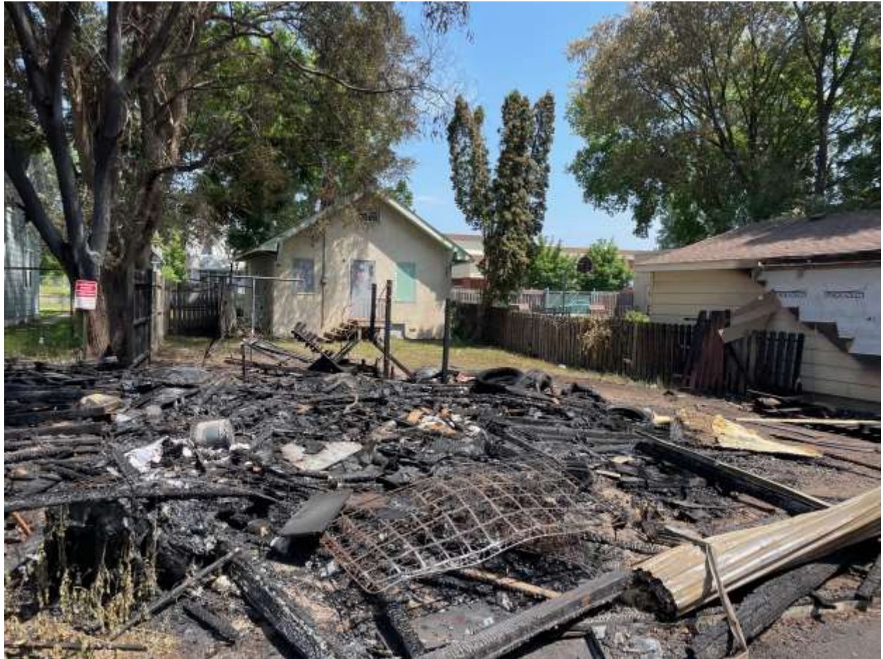
792 Rose Ave E. Garage fire 6/28/23
