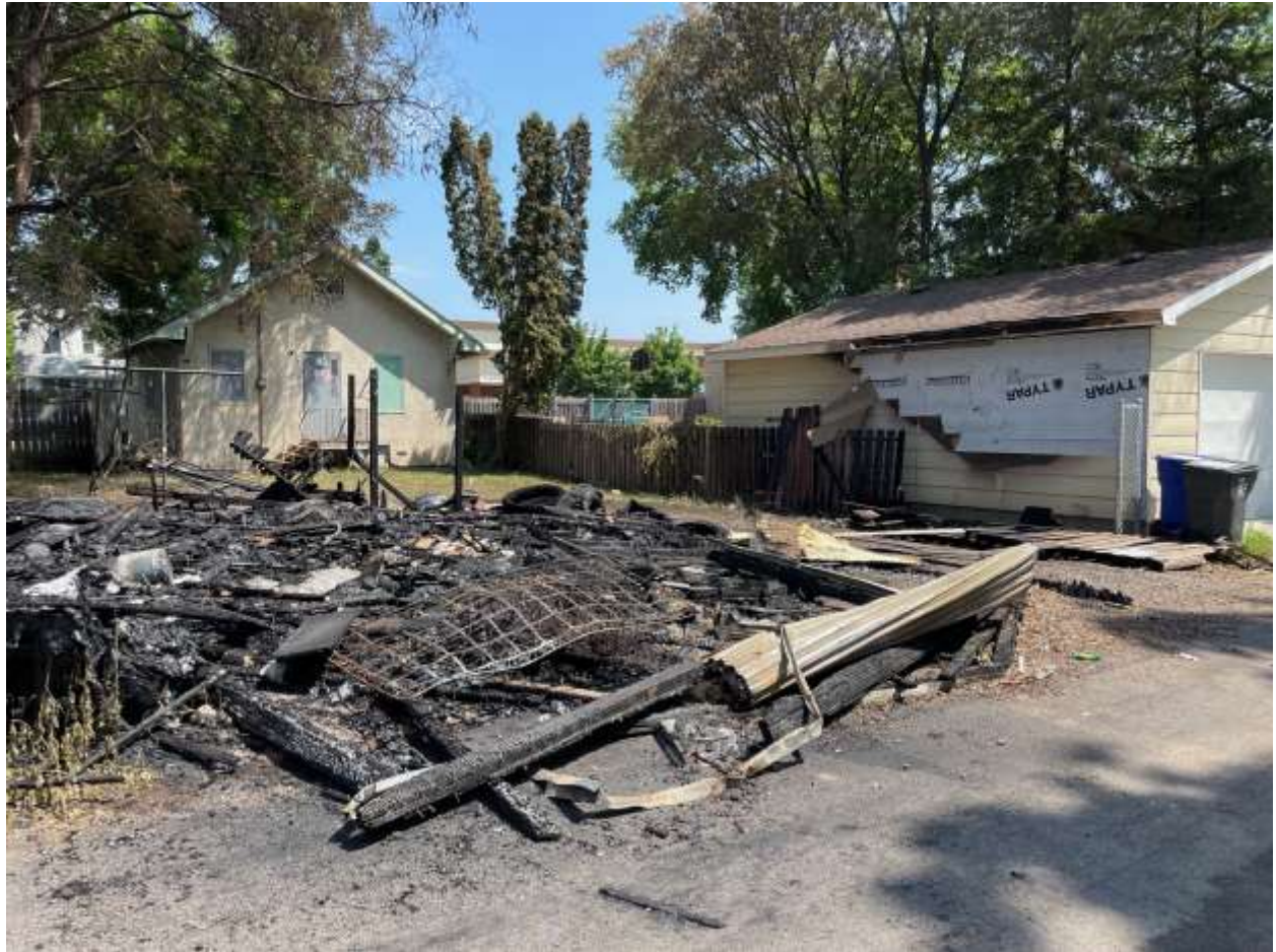
792 Rose Ave E. Garage fire 6/28/23
