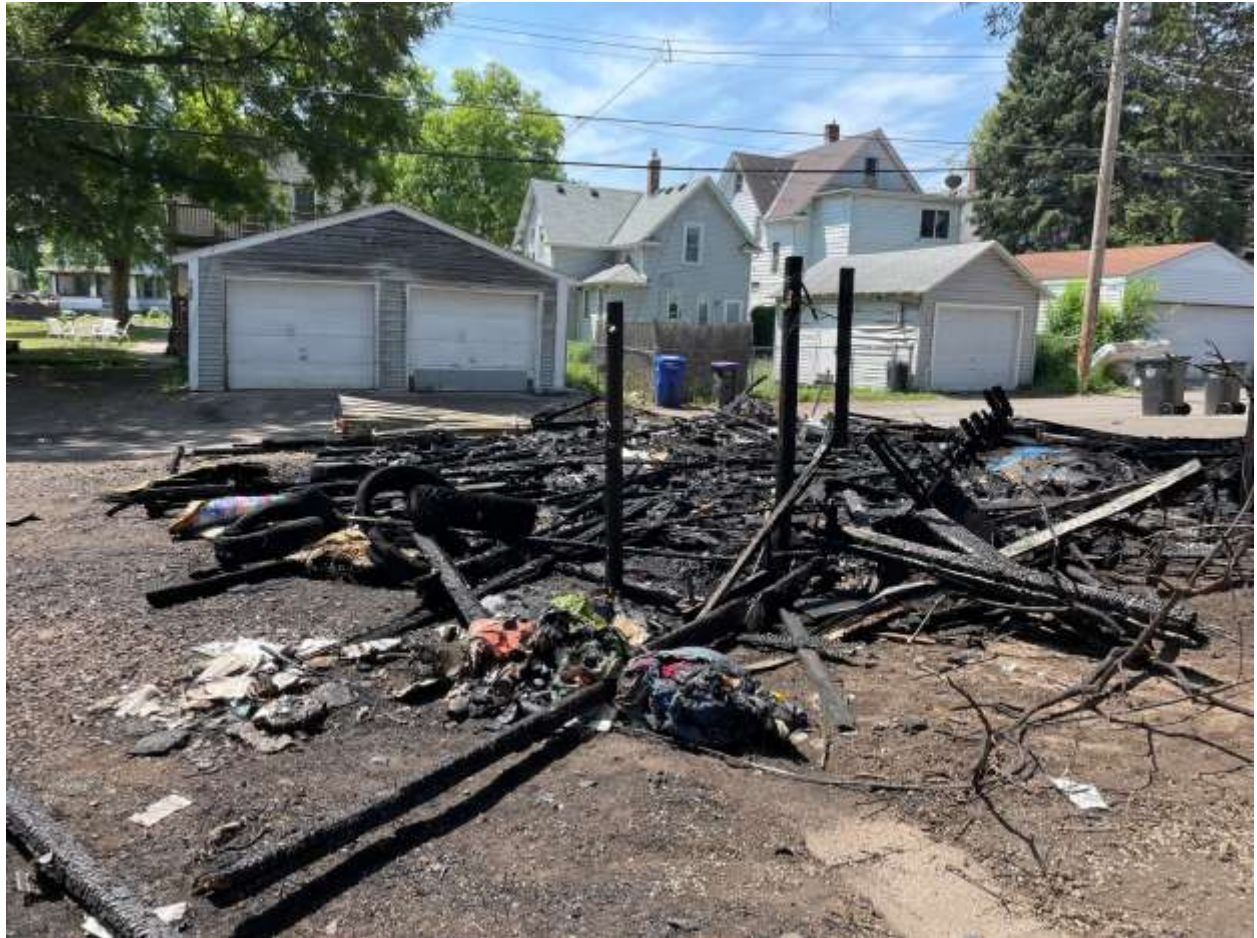
792 Rose Ave E. Garage fire 6/28/23
